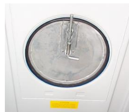
Figure 9.11 Roof hatch internal lock
