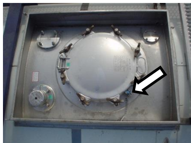
Figure 9.14 Manway hatch seal
